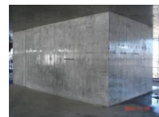
A column and wall built with recycled aggregate concrete
