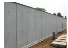
Retaining wall built with recycled aggregate concrete
